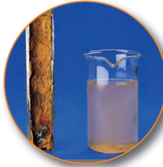
Before: Pitting, rust and brown water
